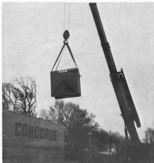
The new equipment about to be lowered through a skylight into the new filmset department.
